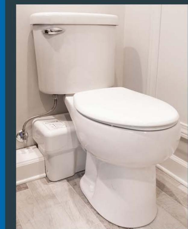
No need to dig into your concrete basement floor. A MACERATING TOILET will get the discharge out to your main sewer line- you can even ADD A SHOWER AND SINK to the pump!
